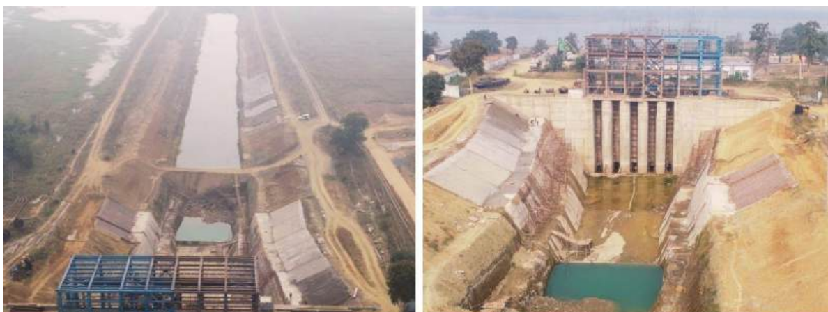
Construction of Check Dam and Water Pump House for Water Conservation, Forebay, Transition Zone and Intake channel, Internal Road & Drain etc, for CW and Make Up Water System
